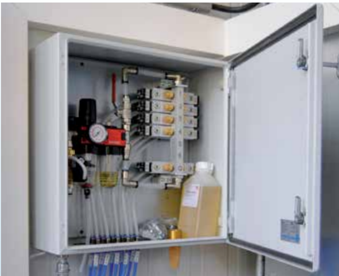
Pneumatic switch box
