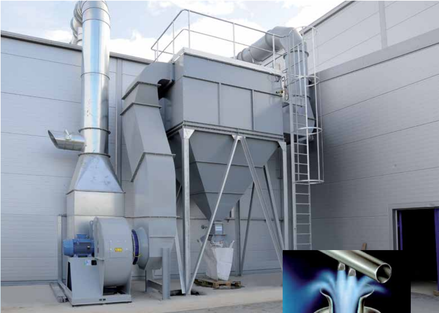
Jet cartridge filter 20,000 m 3 /h with big bag packaging, silencer and radial ventilator
